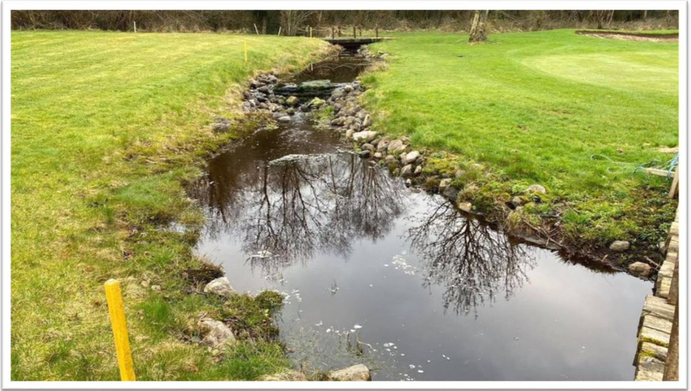
The stream on the left of the bridge on the 5 th hole has been cleared
