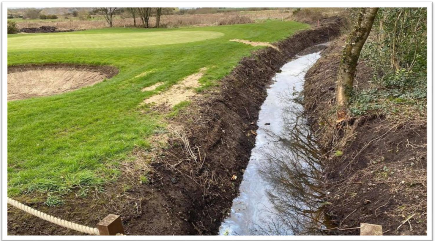
The greenside drain on the 12 th Hole has been cleared
